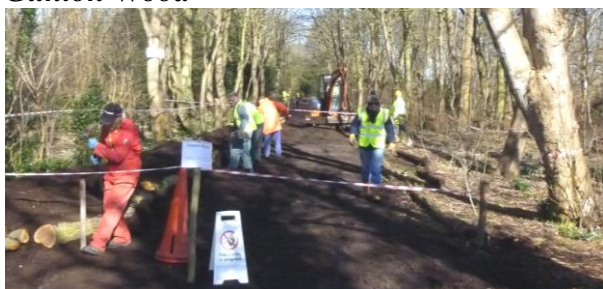
Working on the main footpath
