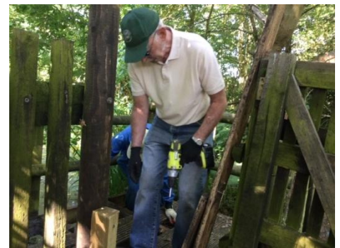
Dismantling the rotten platform
