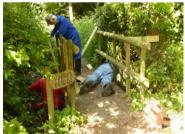
We had a report that the hand rail on Vinnie's bridge was wobbly, so a group of men set about repairing it, but soon found that the posts had rotted, so they were also replaced. An inspection of Freeman's bridge showed that it also needed some repairs. Both bridges are now safe and secure.
