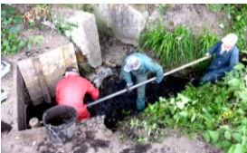
Culvert clean-out
